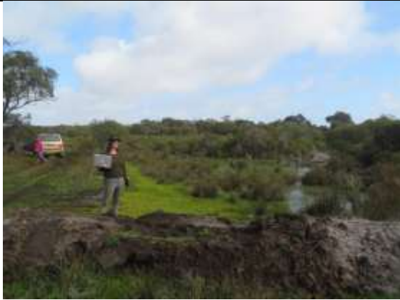
Site H8 & H7: Earthworks undertaken to try and retain water on-site in Melaleuca wetland.
