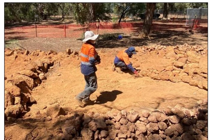
Mystine and Mitch laying rocks for water control at Kalamunda
