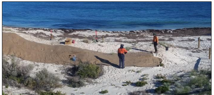
Jan and Perri laying erosion matting in Cockburn
